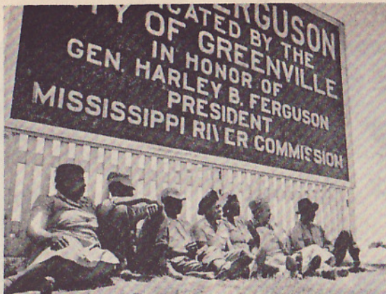
10. The sign gave just enough shade for these folks to watch the levee in comfort. Lake Ferguson was really an old unused riverbed.
