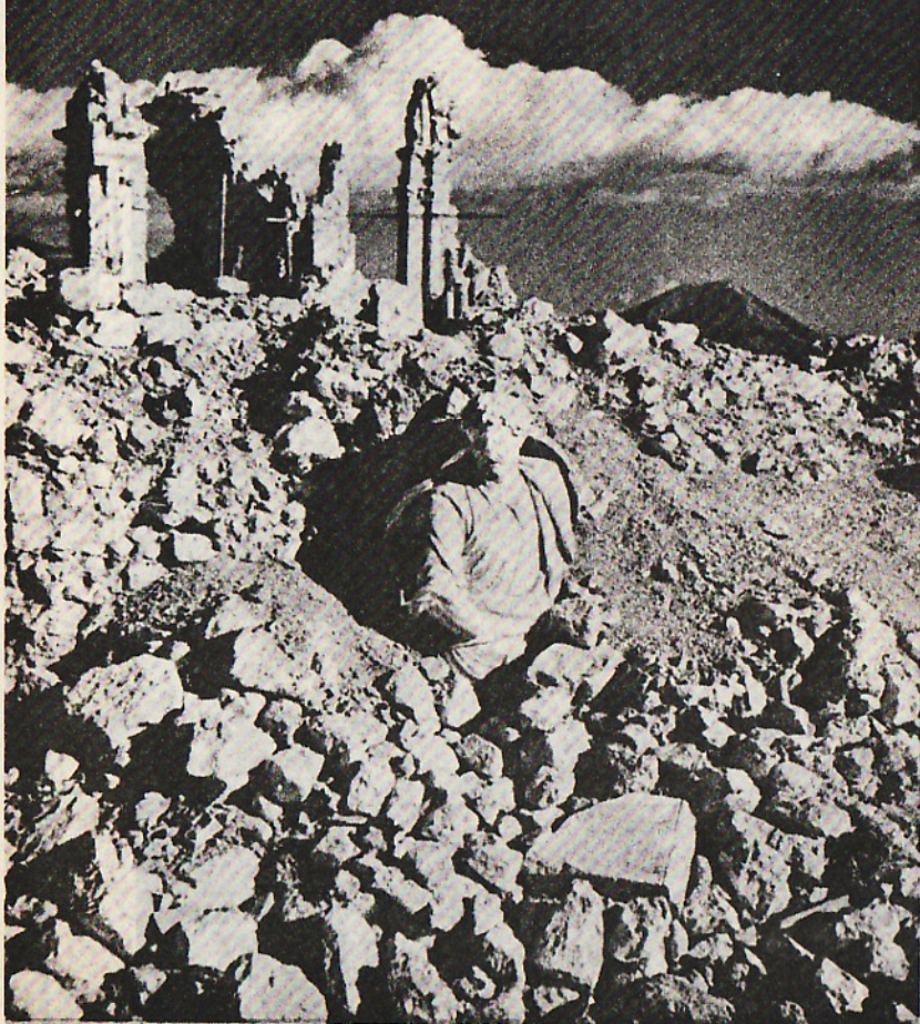
In the Benedictine Abbey of Montecassino a bust lies on a pile of rubble. The Nazis first used the Abbey as an observation post, and an ammunition dump was found near its walls. Later, after Allied bombing, they had gun positions there.
