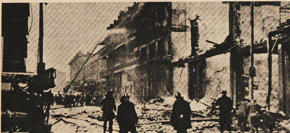
DISASTER. AFTER AN ALL-NIGHT BLAZE, FIREMEN STILL HAD TO POUR WATER INTO THE GUTTED BUILDINGS OF THE BUSINESS SECTION OF DUQUESNE, PA. THE FIRE STARTED IN A FURNITURE STORE AND DESTROYED 12 BUILDINGS, KILLED A MAN AND LEFT 150 HOMELESS.
