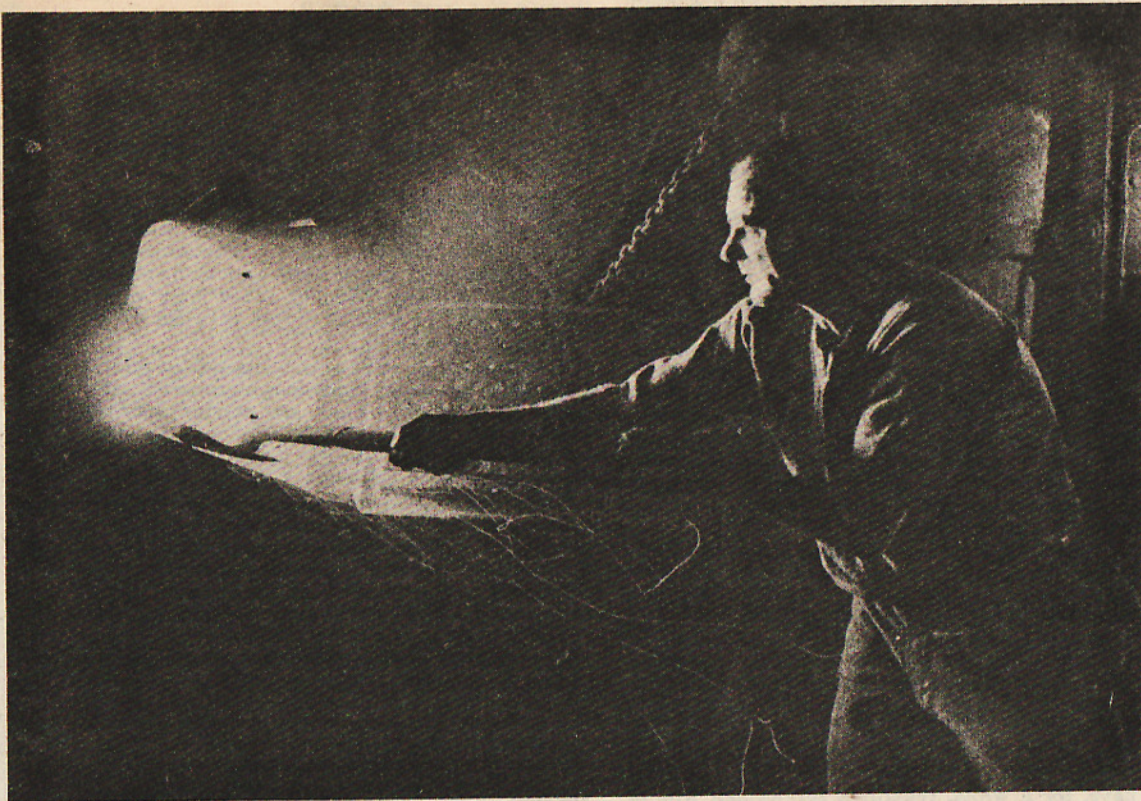
Deep in the bowels of the tug, tremendous power must be generated 24 hours a day.
