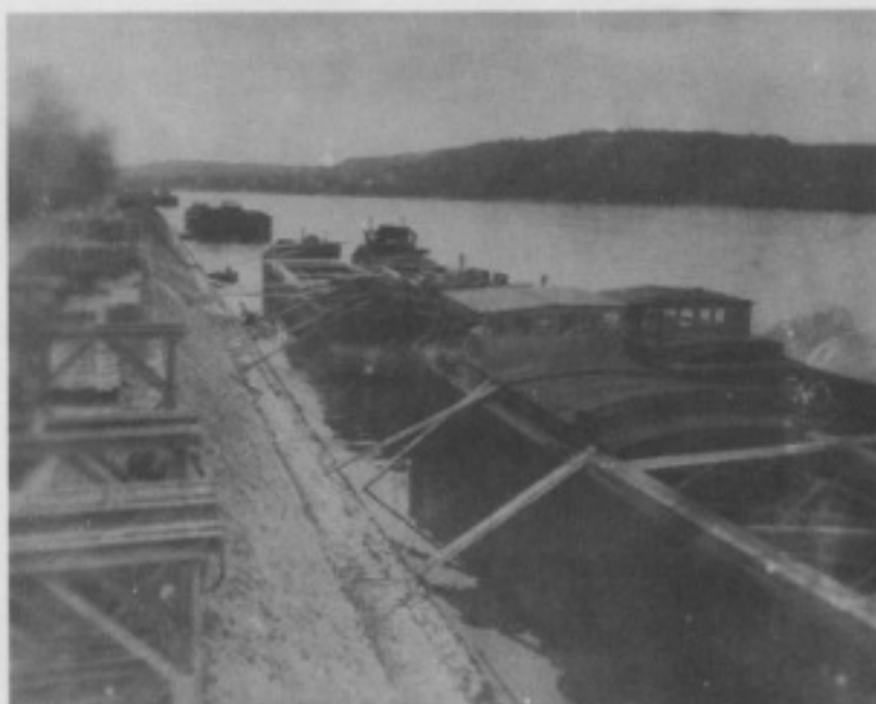
Fig. 4. FLOATING BAY PIERS PRIOR TO LAUNCHING OF TRUSS
