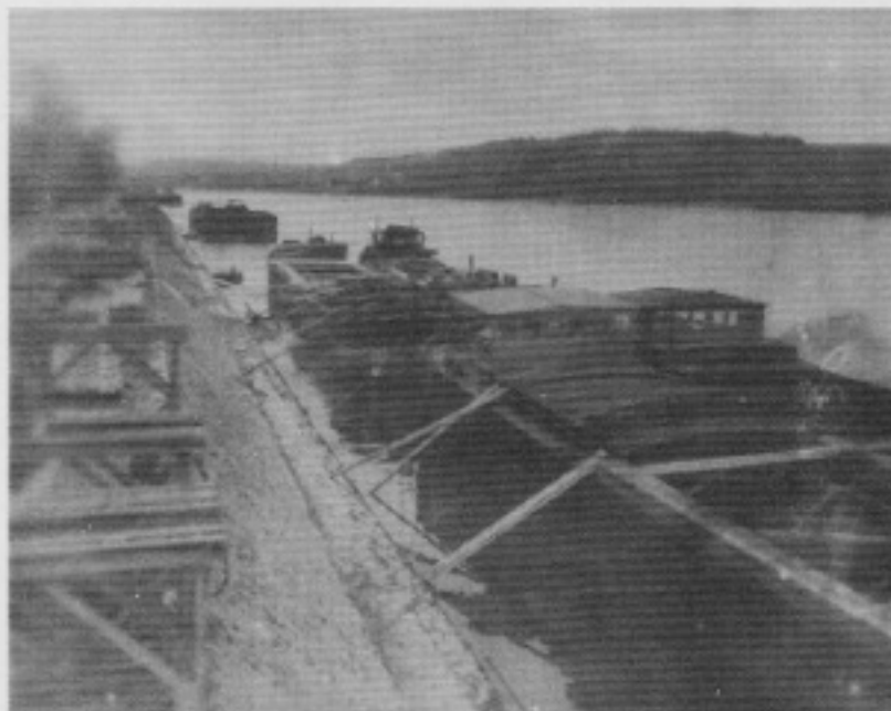
Fig. 4. FLOATING BAY PIERS PRIOR TO LAUNCHING OF TRUSS
