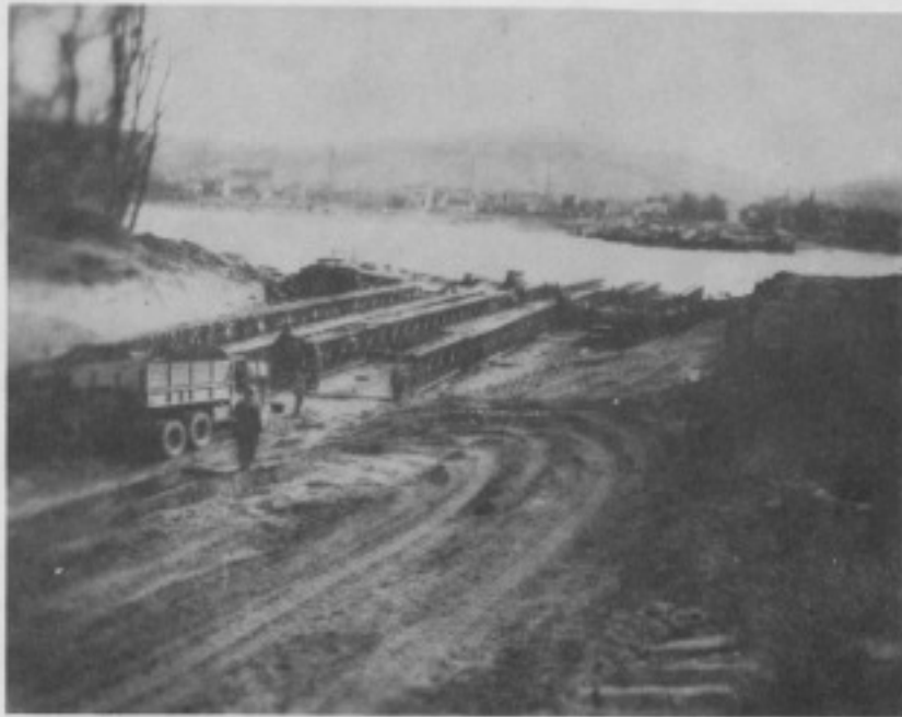
Fig. 25. SHORE AND RIVER LANDING BAYS CONSTRUCTED TOGETHER
