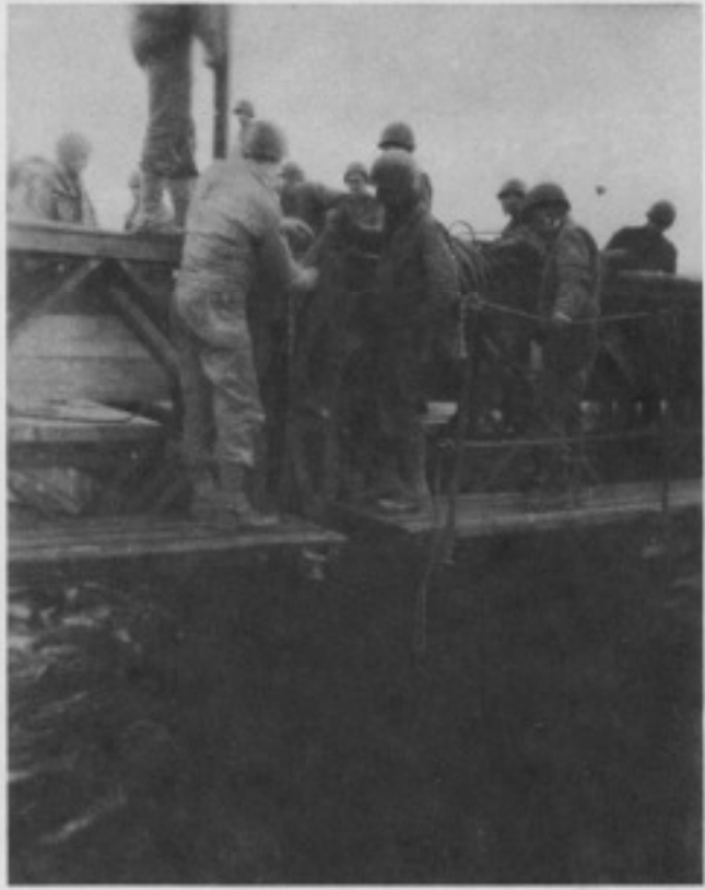
Fig. 39. REMOVING CHAIN HOISTS FOLLOWING CONNECTION OF TWO BAYS OF BRIDGE
