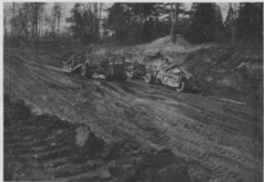
Fig. 27. CARRYALL PANS AT WORK ON WEST APPROACH
