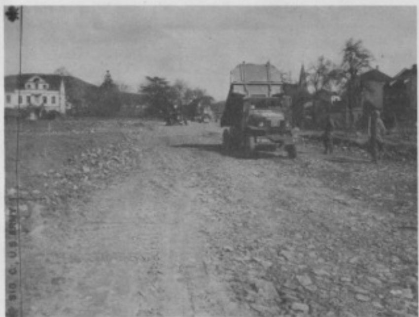
Fig. 32. PLACING 1 1/2 INCH WEARING COURSE OVER BASE COURSE ON EAST APPROACH
