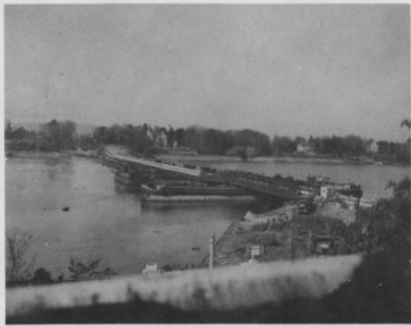
Fig. 36. FULL VIEW OF BRIDGE SHOWING GUY AND ANCHOR LINES
