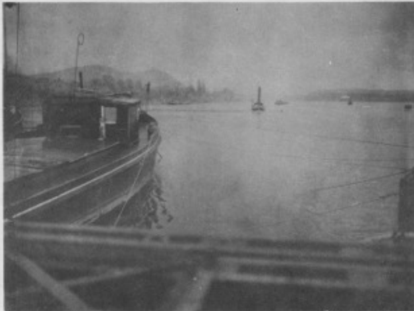
Fig. 37. VIEW FROM BRIDGE LOOKING UPSTREAM SHOWING TIE CABLES, ANCHOR CABLES, AND ANCHOR TUG WHICH RESTS IN SHALLOW WATER ABOVE THE JETTY
