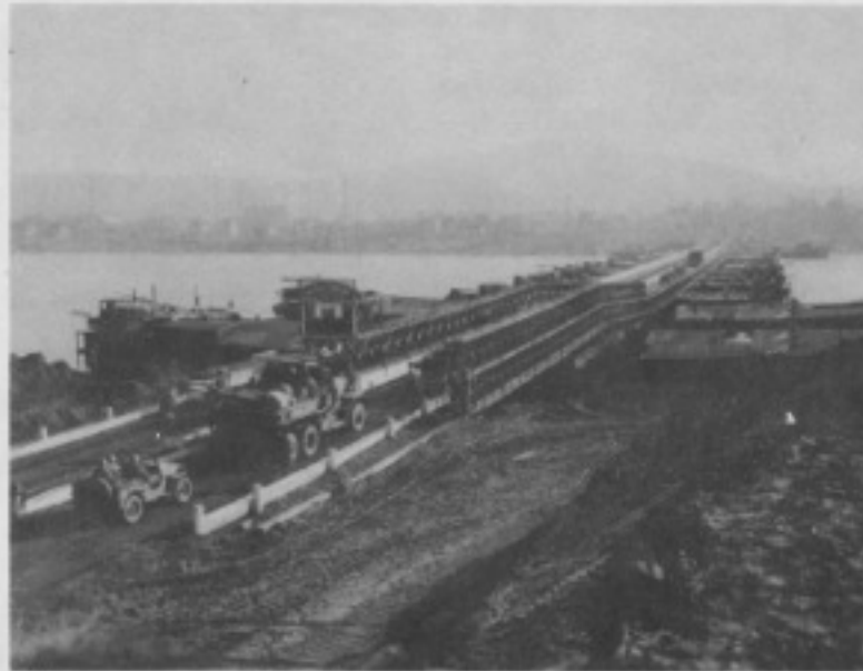
Fig. 15. GENERAL VIEW OF BRIDGE FROM WEST BANK
