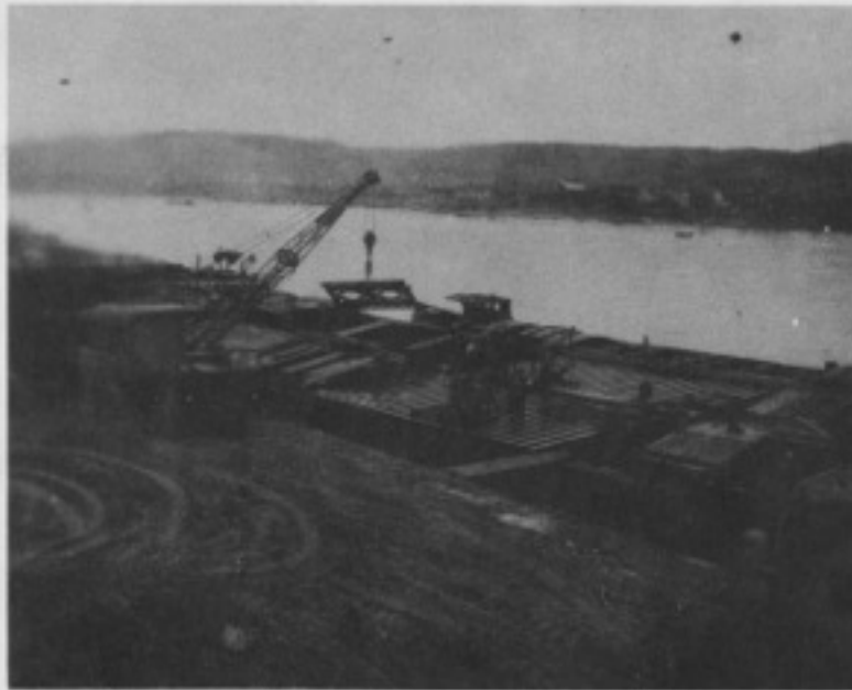
Fig. 10. LANDING BAY PIER AS CONSTRUCTION OF END FLOATING BAY STARTS
