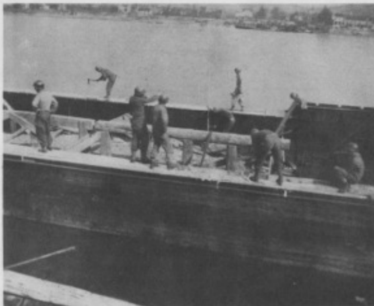
Fig. 8. I-BEAM CRIBBING OF WEST SHORE INTERMEDIATE LANDING BAY PIER
