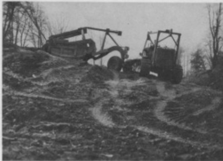
Fig. 29. CARRYALL PAN IN OPERATION
