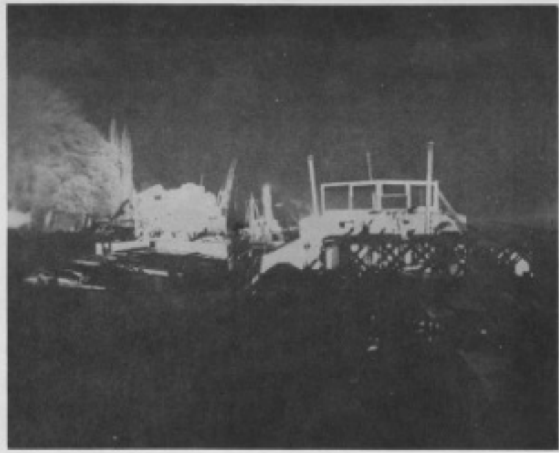
Fig. 16. NIGHT CONSTRUCTION WITH ARTIFICIAL ILLUMINATION
