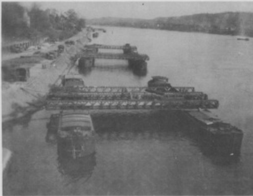
Fig. 3. FLOATING BAYS NEARING COMPLETION
