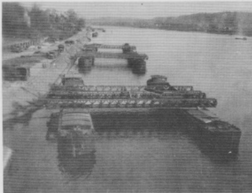
Fig. 3. FLOATING BAYS NEARING COMPLETION
