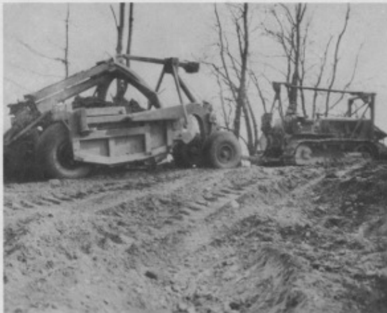
Fig. 30 LOADED CARRYALL PAN LEAVING CUT
