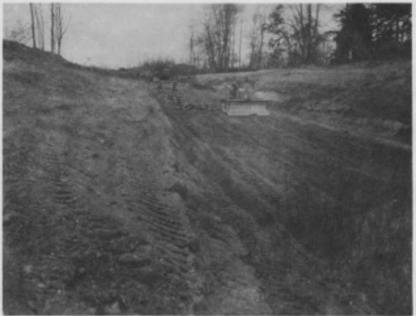
Fig. 28. BASE COURSE BEING PLACED BEFORE COMPLETION OF EXCAVATION
