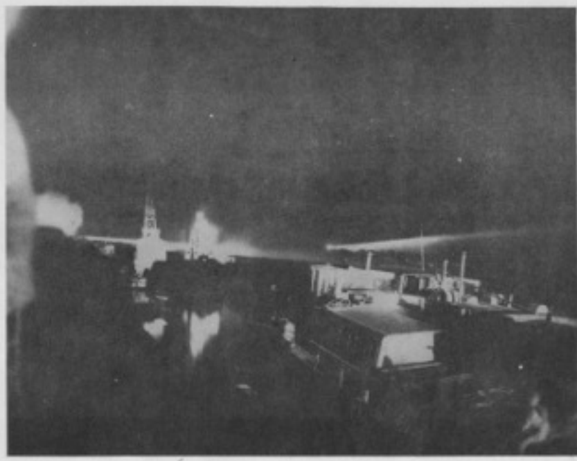
Fig. 17. ARTIFICIAL ILLUMINATION FOR NIGHT CONSTRUCTION
