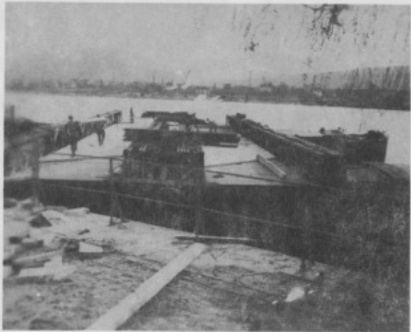
Fig. 43. INSTALLATION OF DIAGONAL TREAD
