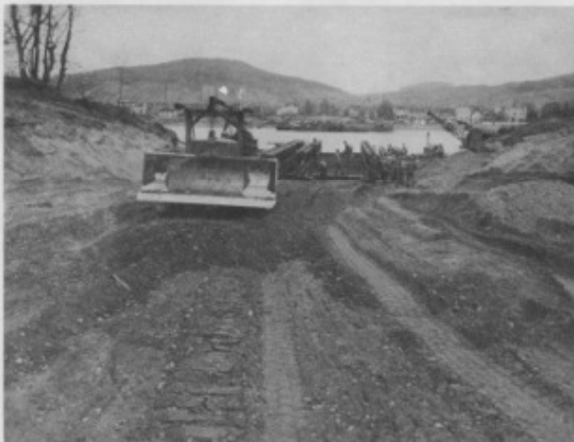
Fig. 26. GRADING AT WEST APPROACH. LANDING BAYS UNDER CONSTRUCTION IN BACKGROUND.
