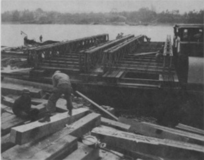
Fig. 5. END FLOATING BAY BEING LAUNCHED. NOTE BEARING ON BOTTOM OF CONNECTING POSTS
