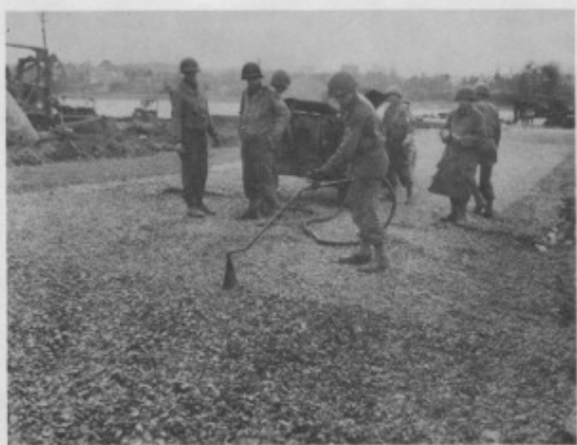
Fig. 33. PRIMER COAT OF TAR BEING APPLIED TO EAST APPROACH
