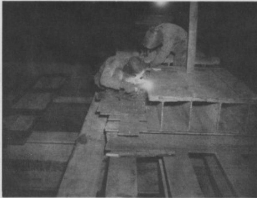
Fig. 8. I-BEAM CRIBBING OF WEST SHORE INTERMEDIATE LANDING BAY PIER
