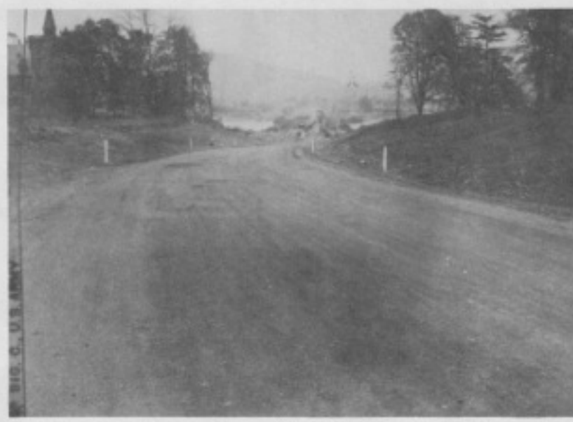
Fig. 34. COMPLETED WEST SHORE APPROACH
