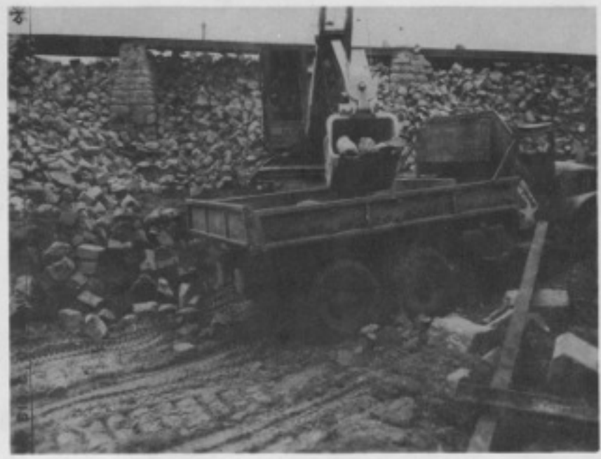
Fig. 31. LOADING BASE COURSE MATERIAL
