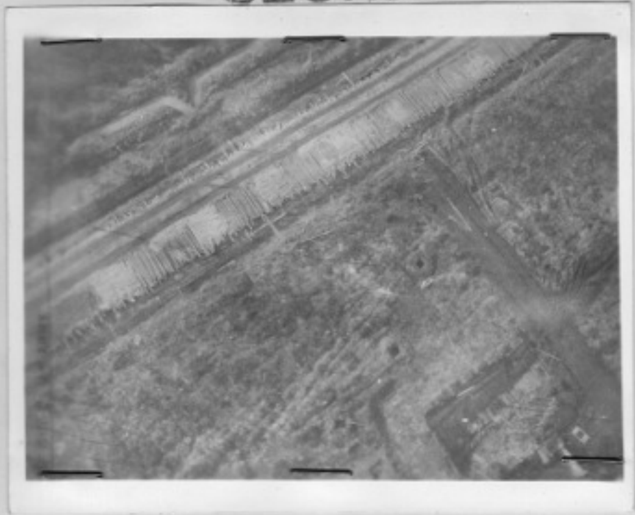
N-31 EUPEN TO MONSCHAU (From the Air) CORDUROY, ONE LANE COMPLETE, LOGS DISTRIBUTED FOR 2ND LANE; 207 ENGR C BN.
