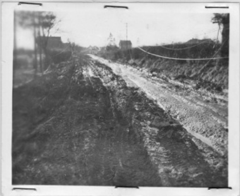
N-51 EUPEN TO MONSCHAU ROAD AFTER FAILURE
