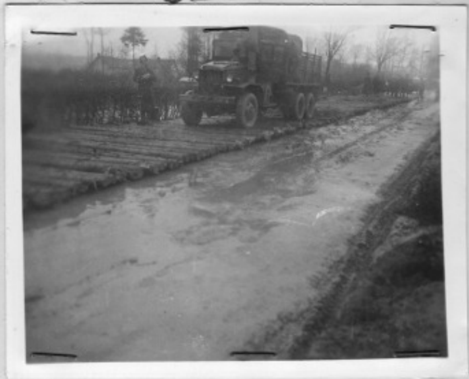
N-31 EUPEN TO MONSCHAU SHOWING CORDUROY LAID FOR ONE LANE WITH NO ROCK - 207TH ENGINEER COMBAT BN
