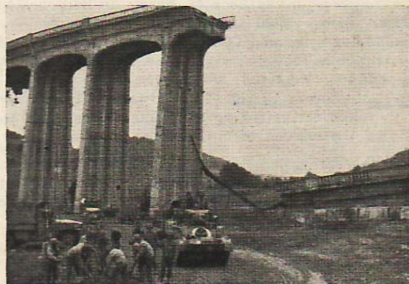
Vehicles of the 87th Cav Rcn Squadron (Mez) pass a demolished bridge near METZ, France, over a road being repaired by engineers.
