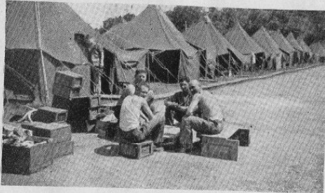
A BATTERY STREET AT BLANDFORD
