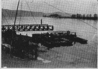
SCENE'S OF THE CONSTRUCTION OF A BAILEY BRIDGE ACCROSS THE RHINE WHILE A "D" BATTERY M-15 COVERS THE ENGINEERS
