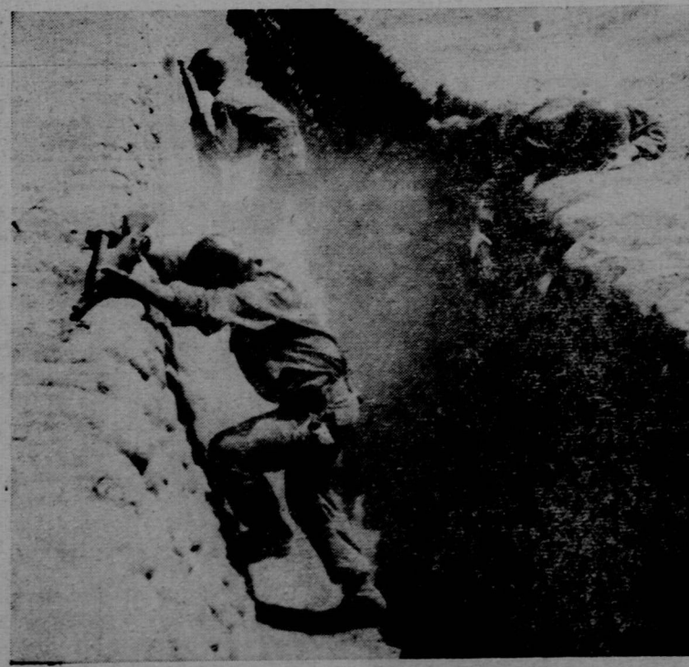
IN AND OUT OF TRENCHES REQUIRES FAST FOOTWORK.
