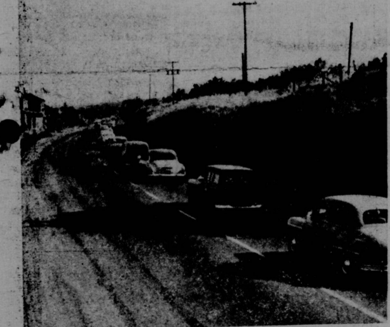
TRAFFIC VOLUME —is over 12,000 vehicles per 24-hour period on the overcrowded two lane highway from Camp Roberts.
