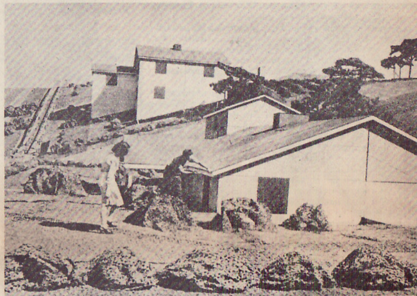
ROOFTOP VILLAGE. These are just a few of the fifty-three artificial houses built on top of Boeing's B-29 plant in Seattle to hide it from possible enemy air raids. From the sky you can't see that there are no bottom floors.
