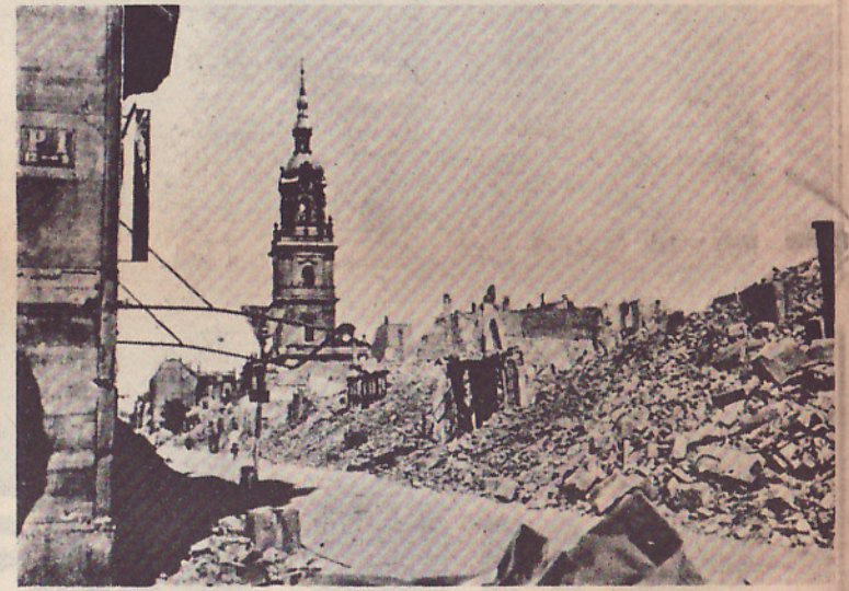
The City Hall Tower stands yet, but the main street on both sides of the building is stacked with piles of stone.
