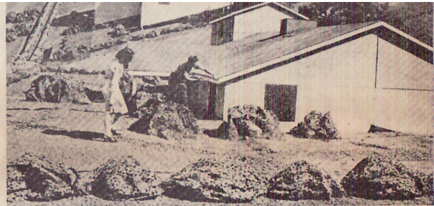
ROOFTOP VILLAGE. These are just a few of the fifty-three artificial houses built on top of Boeing's B-29 plant in Seattle to hide it from possible enemy air raids. From the sky you can't see that there are no bottom floors.
