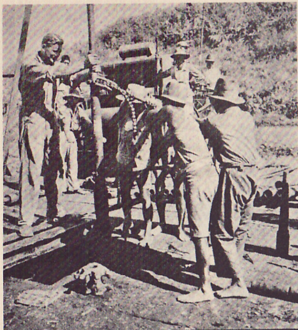
Dutch sergeant supervises Indonesian oil men testing to see what is plugging up the well.
