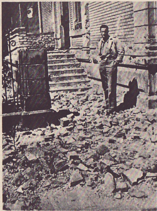
The iron gate in front of the house is gone, per- haps for scrap. My picture was taken here.
