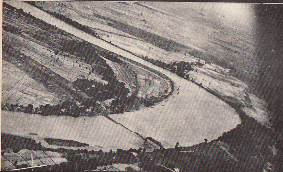
As the bombers flew back to their field they left the Daga bridge with three of its four trestles smashed.
