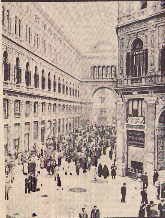
The Galleria is the Radio City of Naples. Glass roof is wrecked but crowds still gather at noon.
